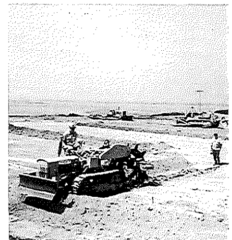
The beginning of our new building project
